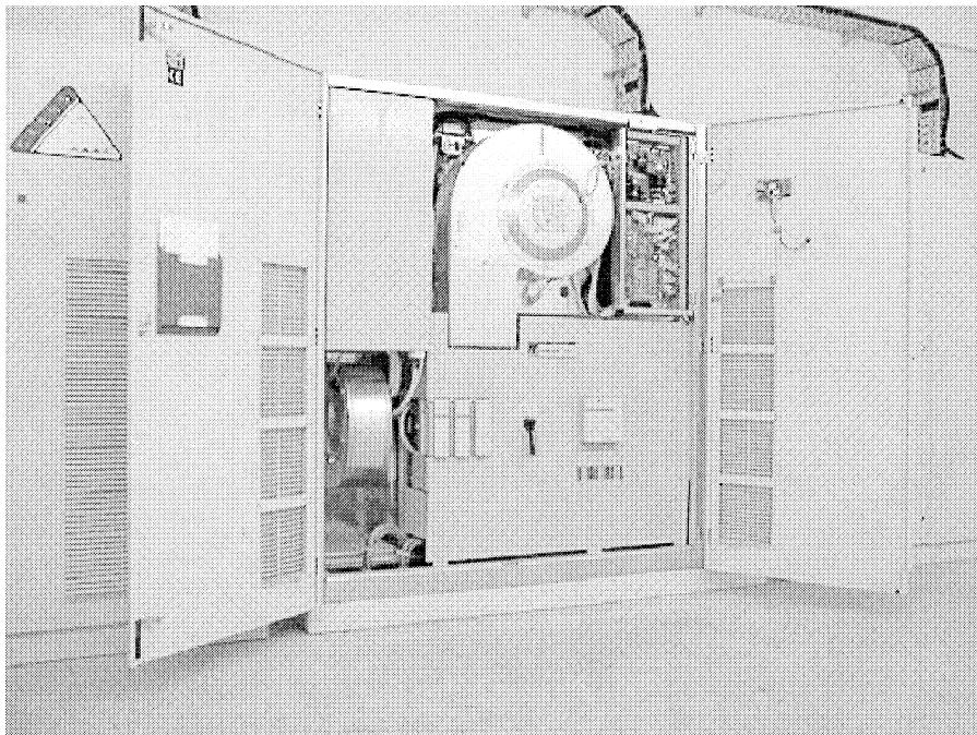
Fig. 9. Detail picture of a 400 kW-rated UPCS power converter.
